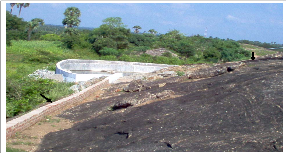
Rainwater harvesting schemes implemented by Private institutions in Palghat ( photograph taken during RHS – Palghat)
