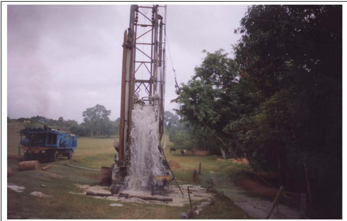
Drilling under progress with high discharge at Nagarur in Trivandrum, Kerala
