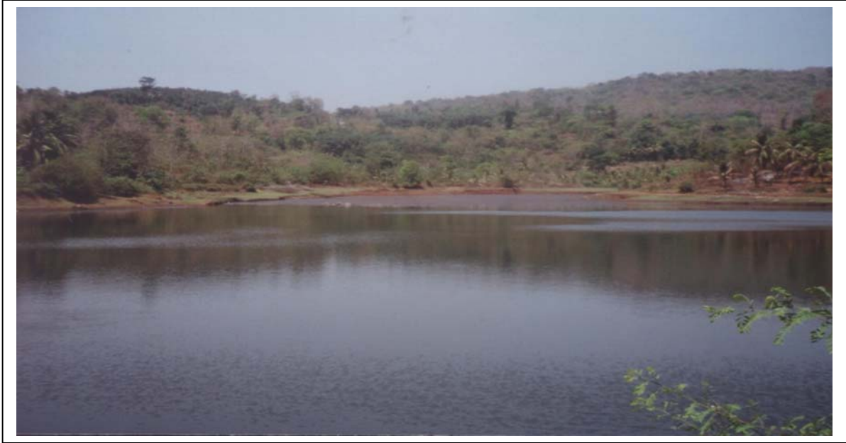
A check dam constructed along the slope atop of a hill at Kachitodu near Pongamodu, Kerala
