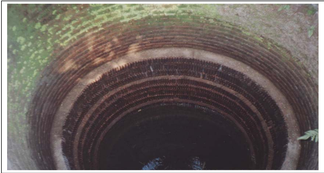
A dug well section showing vertical lining of roof tiles at bottom near Trichur, Kerala
