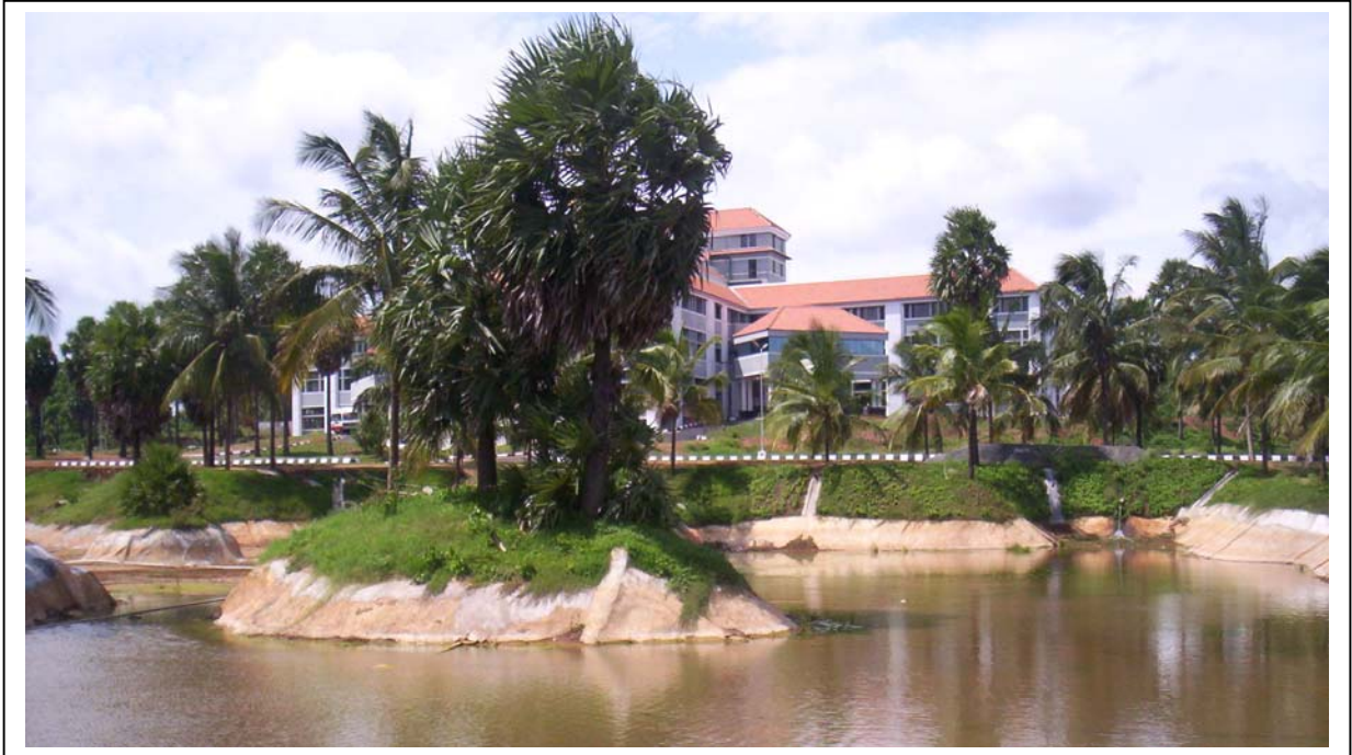
Rainwater harvesting schemes implemented by Private institutions ( Ahliya Hospital) in Palghat district(during RHS – Palghat)
